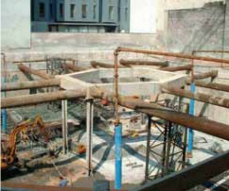
Kurfürstendamm, Berlin Residential and business premises: Support structure planning of the excavation pit as interior bracing with central ring
