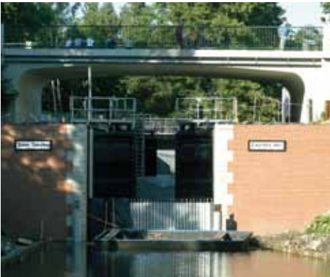
Lock Templin, Brandenburg Replacement taking into account the deformation sensitivity of the rigid frame bridge
