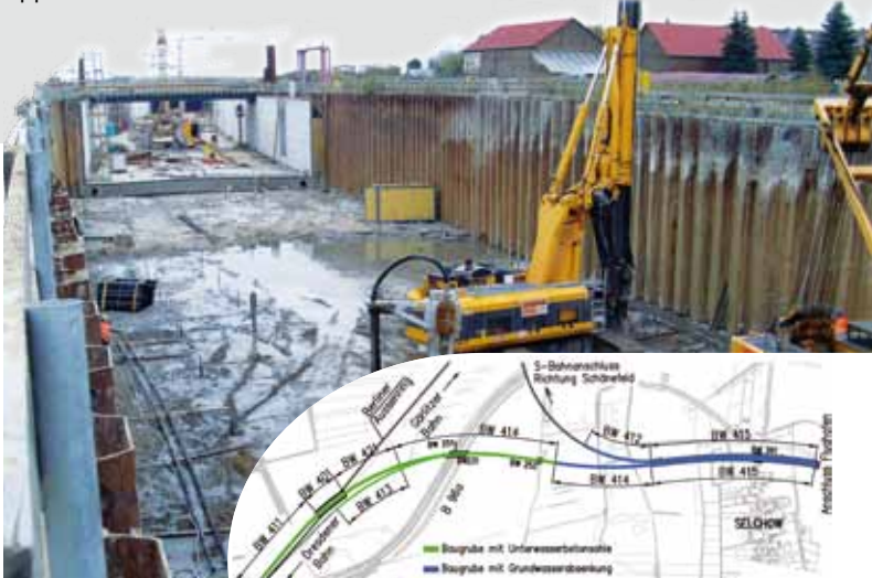
Airport BER, Berlin-Brandenburg Design of excavation pit of the western two-track rail link – routing of the 2.7-km-track mainly as trough route as well as underground in the area of the terminal
