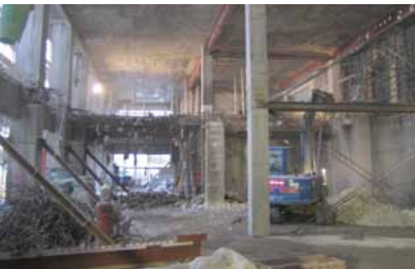
Berolinahaus, Alexanderplatz 1, Berlin Conversion of the listed building from the basement up to the 3 rd floor to a shopping center by enlarging the existing support grid using bracing structures of reinforced concrete and steel composite structures on the 4 th floor
