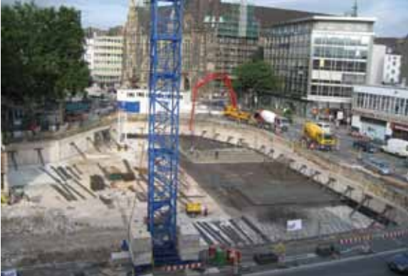
Shopping Center, Wuppertal Support structure planning for demolition and construction of a shopping center while using the existing basement as trench casing and the existing bottom seal for the new locations of the supports
