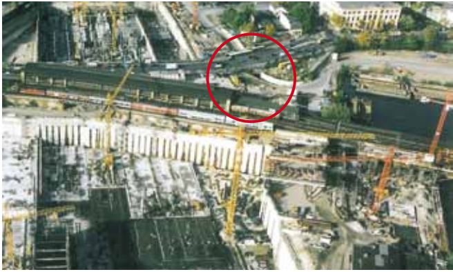
Excavation pit S21 Central Station, Berlin The civil engineering structure consisting of several partial excavation pits of the train line S21 is embedded approx. 18 m in the subsoil with a rear-anchored base
